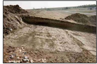
**Concrete and Pan Construction:** Concrete curbs were placed to enclose an approximate 30-foot by 50-foot area. The curbs were extended vertically 6 inches above the subgrade and were 12 inches wide. Soil material was sloped from the subgrade to the top of the curb. A surveyor located the sump pit which was then excavated using a track hoe. The sloped area and subgrade were then smooth rolled to provide a smooth surface for which to place poly-vinyl chloride (PVC) plastic liner.
