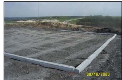
**PVC Liner Installation:** After the subgrade, concrete curbs, and sump pit were constructed, a sheet of factory-welded PVC liner was deployed over each lysimeter base. The PVC panels were pre-fabricated to be 42-feet wide by 60-feet long so the material could overlap the curbs and fit inside the sump. Field welding for adjacent panels was not
