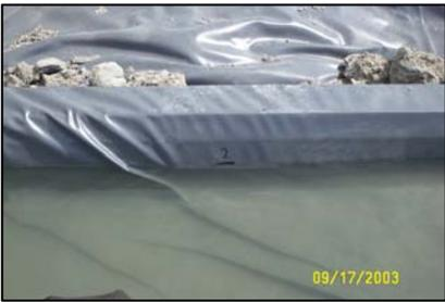
**Geocomposite Drainage Layer Installation:** A 6 ounce per square yard (oz/yd<sup>2</sup>), double-sided geocomposite drainage layer was partially installed over the PVC liner prior to conducting the lysimeter pan leak tests, leaving the sump areas uncovered. The geocomposite placement was
