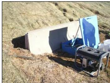
from covering the lysimeter vault. As a result of the settling and pipe shearing, the piping from the lysimeter pan was no longer connected to the lysimeter vault. The jersey barrier was removed and the piping repaired on December 28 and 29, 2004. The jersey barrier was replaced with a section of lighter corrugated metal piping.
